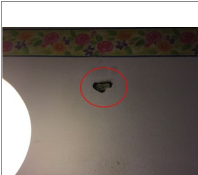
Improper electrical outlet in the kitchen wall.
