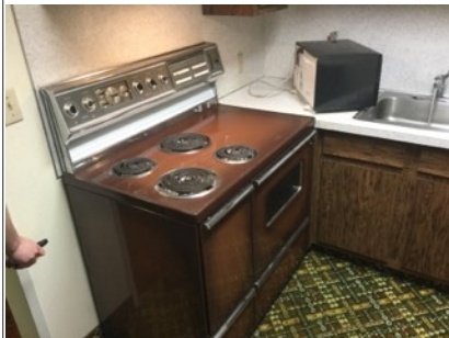
Electric range in basement kitchen was operating
